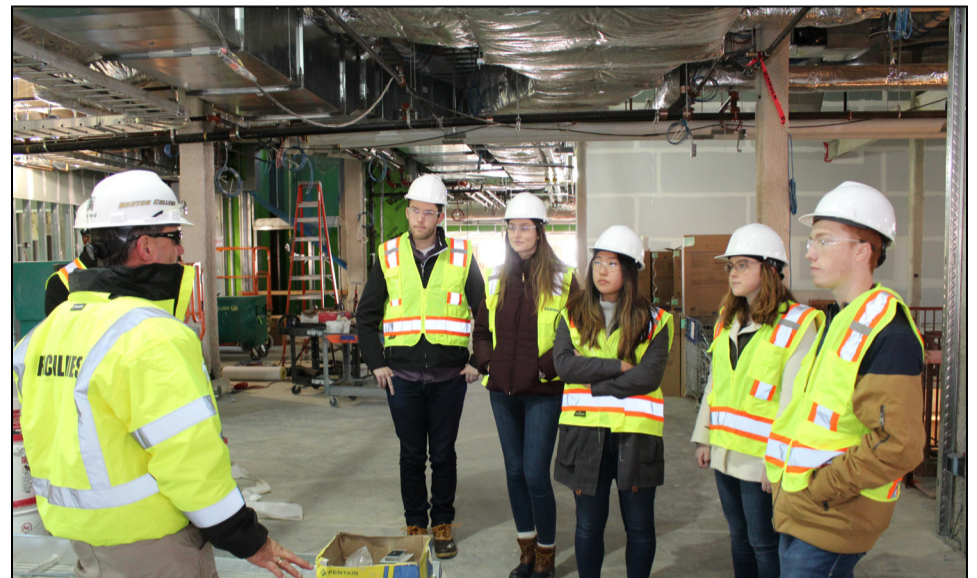
EcoPledge toured the Connell Recreation Center construction site last month.
